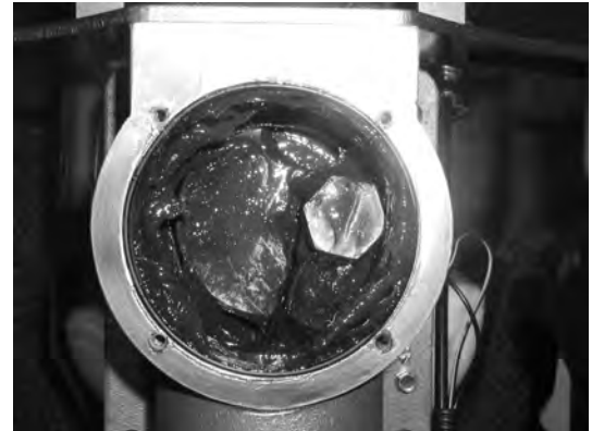
Fig. 2 - Inspect color and amount of grease.
